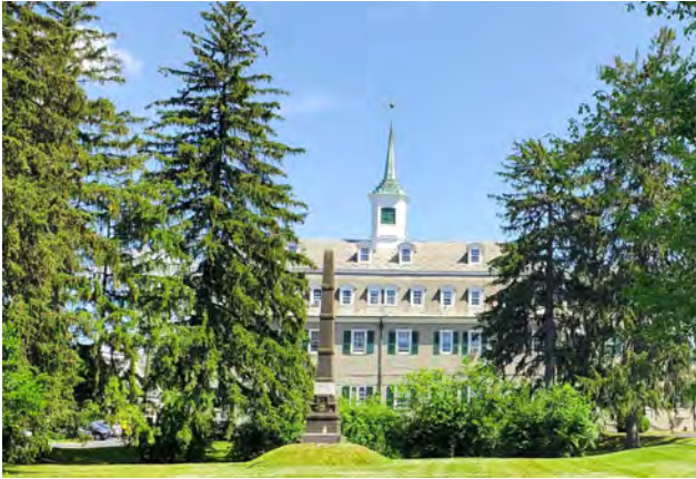
Nazareth Hall Square Manor House - 1756 with Monument
