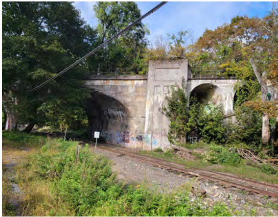
Railroad Cut-off Bridge
