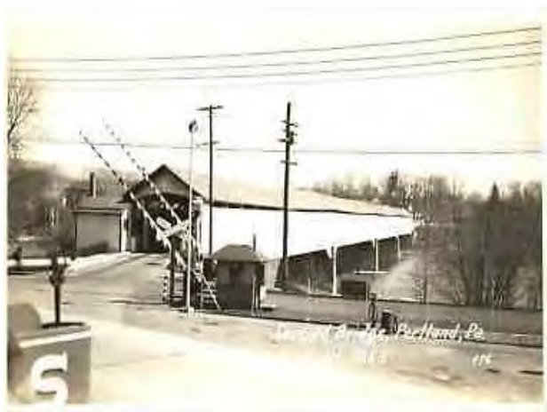
Portland Covered Bridge - 1855
