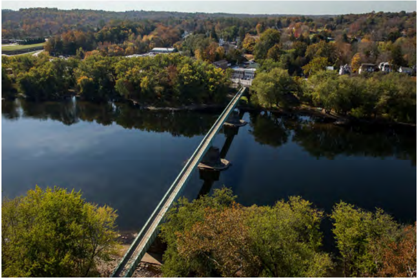
Portland Walking Bridge
