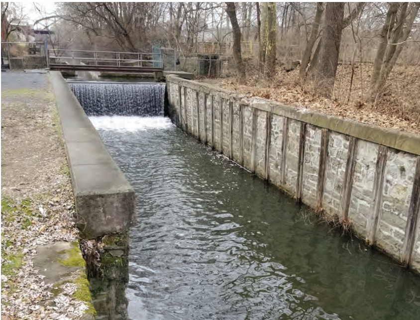
View of Lock 42 - 2023
